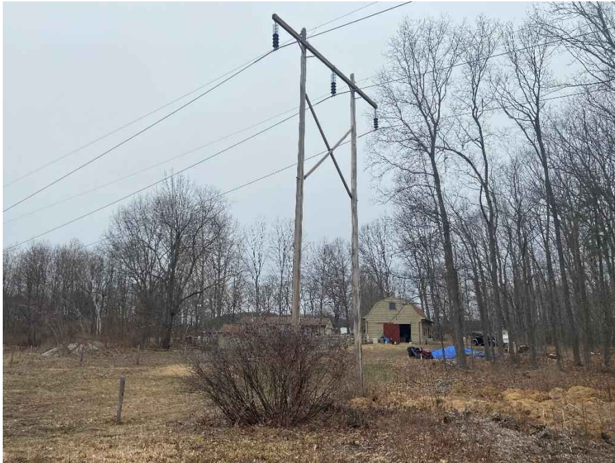
Photograph No. 1: Looking northerly at M183 Structure 3 to be replaced.
