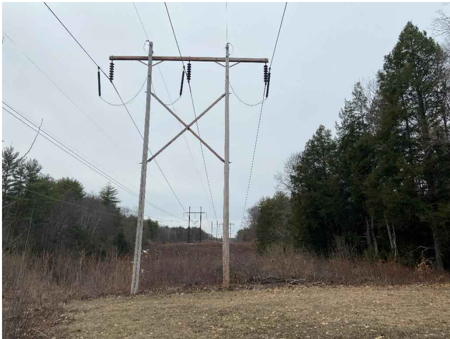
Photograph No. 6: Looking easterly at M183 Structure 3 to be replaced.
