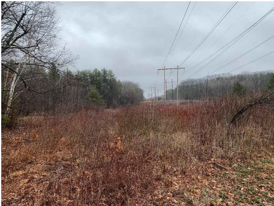
Photograph No. 4: Looking easterly at existing access road from Evans Road to M183 Structure 5 to be replaced.
